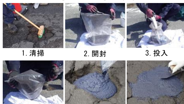
写真-2 補修の流れ Repair procedure
