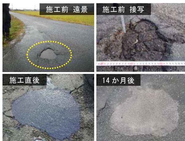
写真-4 穴埋めの適用事例 Construction examples of pothole patching
