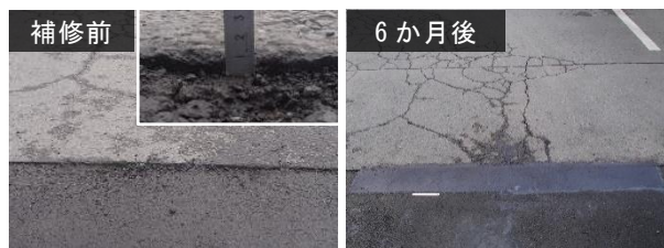
写真-5 段差すりつけの適用事例 Construction example of partially treatment
